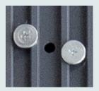
2 lugs at each of the four fixing points per side.
