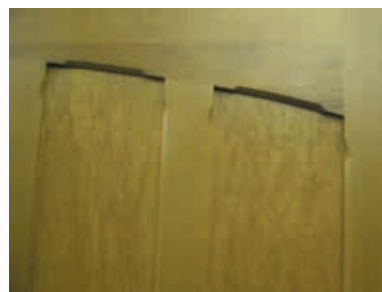
Panel detail of plywood panelled doors with cedar facings showing stopped chamfer profile
