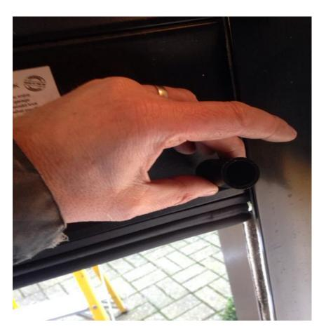
Take the Bottom slat out of the guides, then pull the optical eyes out of the rubber.
