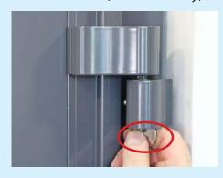
**4.** Insert the door key head and turn to adjust.
