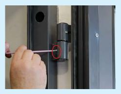
**2.** Open the door, loosen the M6x5 set screw (4mm allen key).
