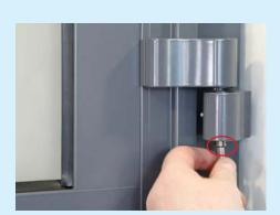
**2.** Close the door and remove the M12 set screw .
