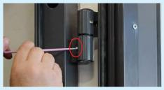
**3.** Open the door, loosen the M6x5 set screw (4mm allen key).
