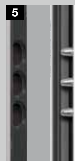
Security bolts on the hinge side
