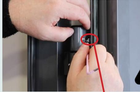
**!** Do not attempt to remove the hinge cover without releasing the set screw. Damage will occur!
