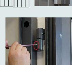
**2.** Open the door, loosen the M6x5 set screw (4mm allen key).
