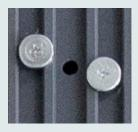
2 lugs at each of the four fixing points per side.
