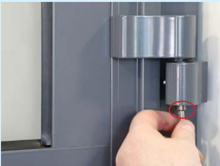
2. Close the door and remove the M12 set screw .
