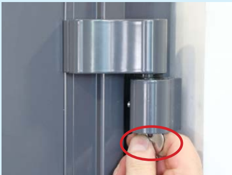
4. Insert the door key head and turn to adjust.
